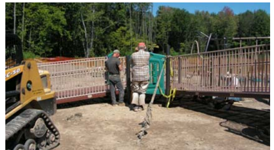
Workers assemble the inclusive playground.
