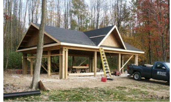
Park district staff builds the pavilion.
