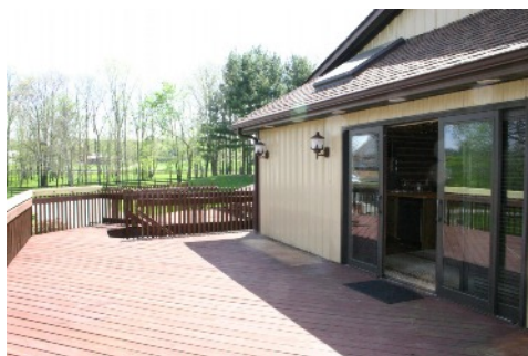
Upstairs deck area
